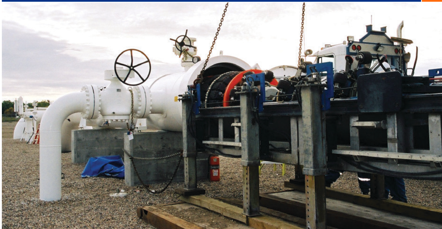
In-line inspection tools are equipped with hundreds of electronic sensors that inspect the quality of the pipeline inside and out to identify even the tiniest crack, flaw or sign of corrosion.
