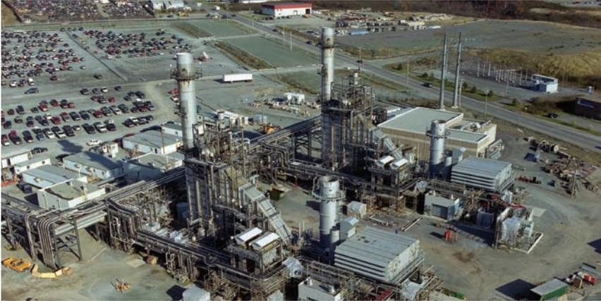
Grandview is an 88 megawatt gas-fired cogeneration power plant that is situated within the Irving Oil Refinery in Saint John, New Brunswick. Under a 20-year tolling arrangement, Irving will provide fuel for the plant and contract for 100 per cent of the plant's heat and electricity output.
